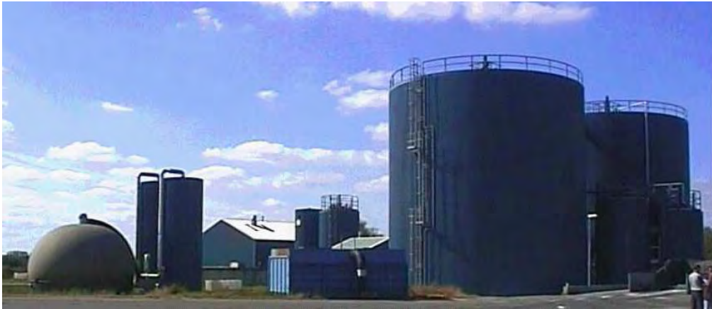
Figure 4 Co-digestion facility for food, manure and other wastes in Denmark – biogas holder left; two digesters right with the two 70 °C sanitisation towers in their shadow.
